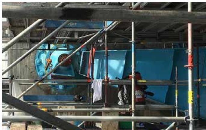
*A sealing side before the gate is installed.*
