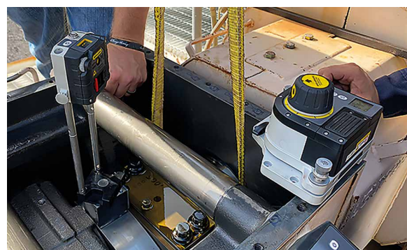
› Checking the main bearing on a compressor.
